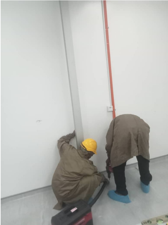
Trunking Job With Our Skill Workers
